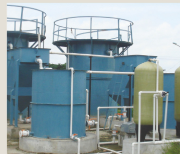
Sewerage Treatment Plant
